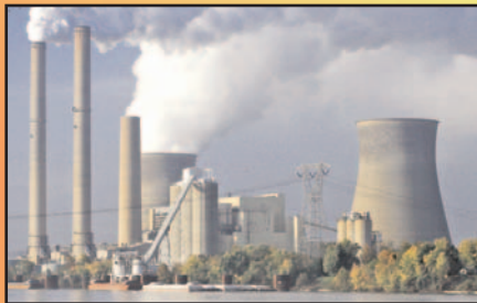
Gavin, Ohio Generating Station photo courtesy of AEP
